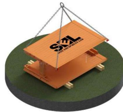
3. Lower opposite panel onto spindles using the 4-Leg chain. Chain hooks to be secured to the handling points at the upper and lower ends of each channel. Secure to spindles as Stage 2. Do not remove slack in the chains until all the spindles are secured.
