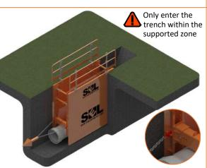
7. Excavate the leading trench and drag the box using two chain legs fixed to the handling points on the cutting edge. Rather than tracking the machine, use the excavators hydraulic arm to drag the box. Once the box is in the next location, adequately backfill
