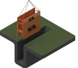
6. Lift box into preformed trench excavated in stable ground. A competent person should assess the ground conditions, ensuring that the ground is temporarily stable and self supporting (see below). A minimum 50mm upstand is recommended.
